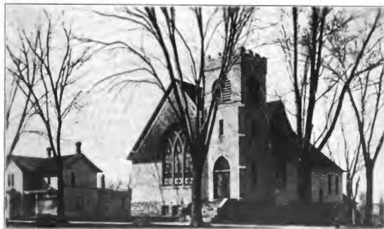
PRESBYTERIAN CHURCH, MECHANICSVILLE
